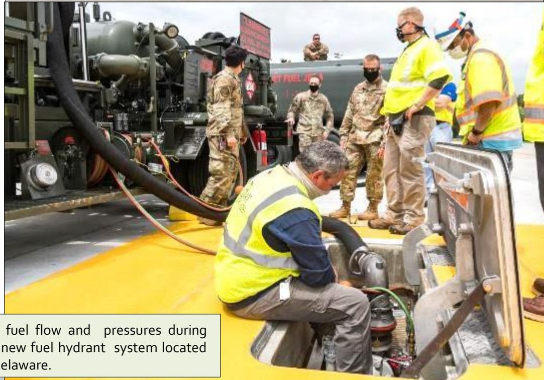
POL-MCX staff observing fuel flow and pressures during operational testing of the new fuel hydrant system located at Dover Air Force Base, Delaware.
