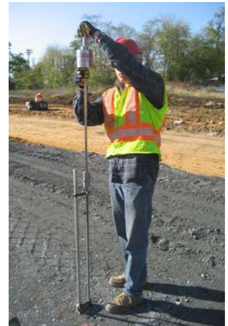
DCP In-situ Strength
