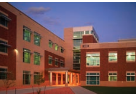
Wilderness Road Complex, Fort Carson, CO, LEED Platinum (from the recent SAME webinar titled "High Performance and Sustainable Building Requirements Unified Facilities Criteria 1-200-02.")
