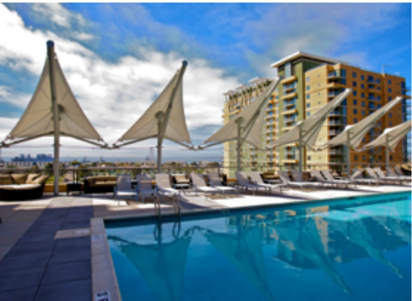
Pacific Beacon Privatized Unaccompanied Housing, San Diego
