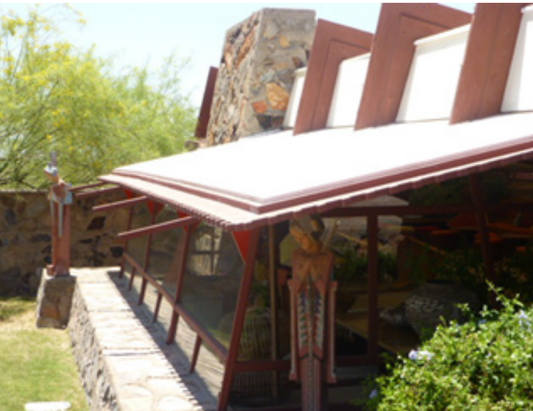
Exterior of living space, Taliesin West
