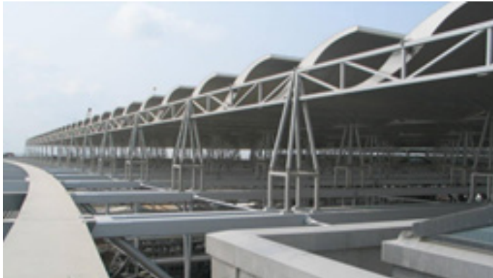
Second Bangkok (Suvarnabhumi) Airport Passenger Terminal Complex – Bangkok, Thailand Murphy/Jahn Architects
