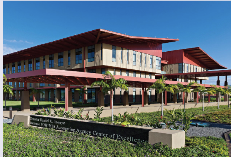
This three story structure was designed to complement and elevate the historic and contemporary architectural character of Hickam Air Force Base. 'Hero's Green' is strategically coupled with the ceremonial Entry Shade Trellis and water feature to balance the functional and ceremonial functions of the facility
