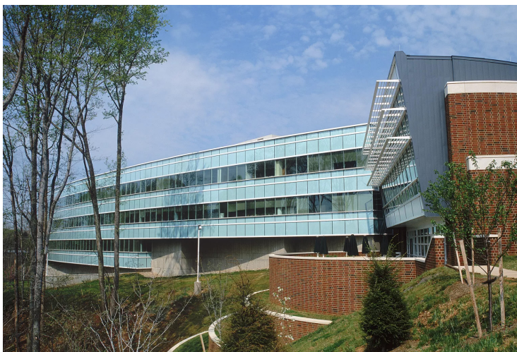
THE NATIONAL GROUND INTELLIGENCE CENTER HEADQUARTERS IN CHARLOTTESVILLE, VA Image courtesy of CallisonRTKL/D Whitcomb
