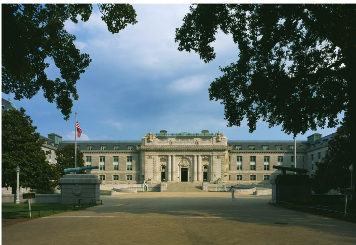
RENOVATED BANCROFT HALL IN ANNAPOLIS, MARYLAND Image courtesy of CallisonRTKL/D Whitcomb
