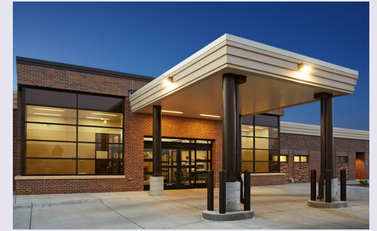
Grand Island Clinic: Renovated front entrance with canopy for drop-off. (Grand Island, NE) • Addition (10,000 SF) & Renovation (22,191 SF). CLH (Prime), Alvine Engineering, InfraStructure, Miller & Associates
