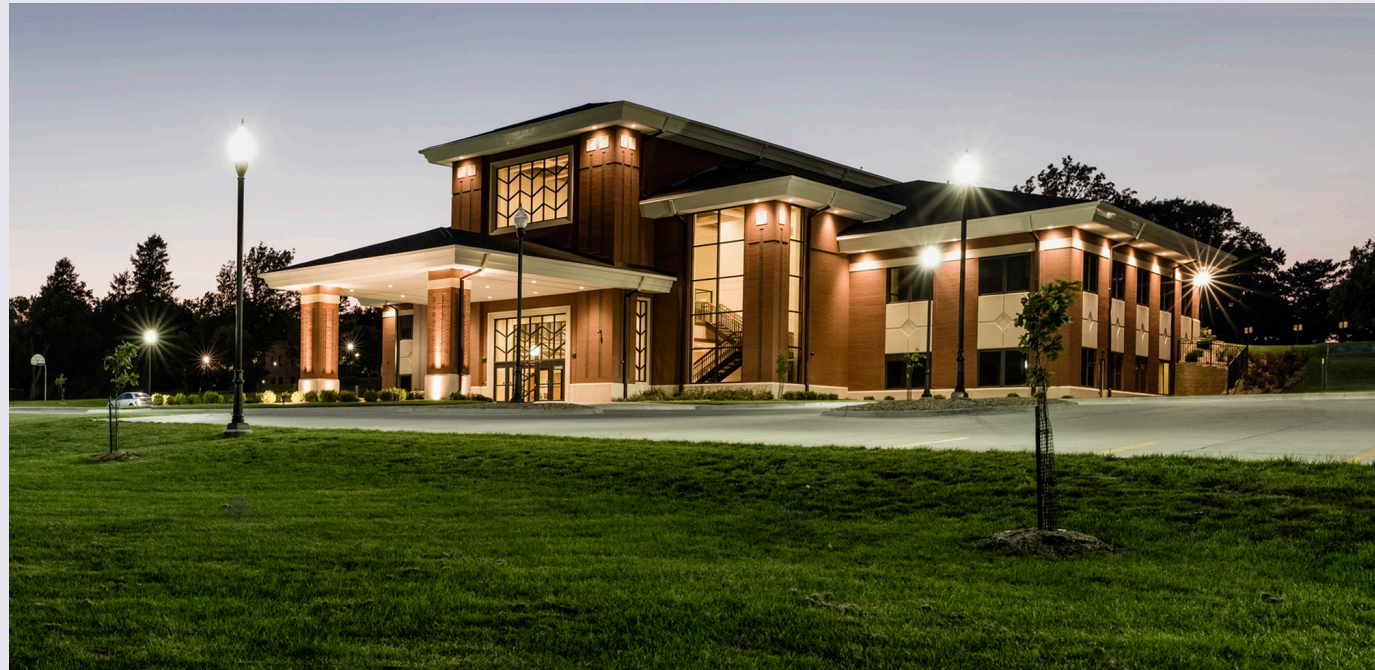
Boys Town Center for Behavioral Health (Boys Town, NE) • New Construction; 40,500 SF. CLH (Prime), Farris Engineering, Ken Lathrum & Associates, Lamp Rynearson & Associates
