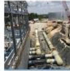
Wet Utilities: 38,000 LF 7 Miles of utilities!
