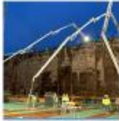
Concrete: 200,000 CY 620 miles of sidewalk!
