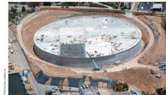
The Earl Thomas Reservoir is nestled in the ground near the main building of San Diego's Alvarado Water Treatment Plant. The reservoir will hold 35 million gal (132 million L) of potable water, making it the largest prestressed-concrete tank in the world. After back-filling and landscaping have been completed, palm trees will grace the reservoir's perimeter and a road will traverse its roof.
