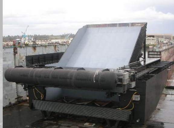
Spillway Weirs – the 'Fish Slide'
