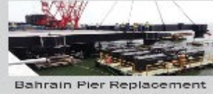
Bahrain Pier Replacement
