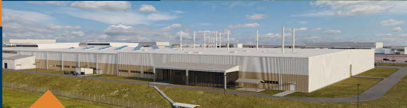
DBB POWERTRAIN PHASES I-IV CCAD NAS Corpus Christi, TX – NAVFAC Southeast Const. Cost $234M
