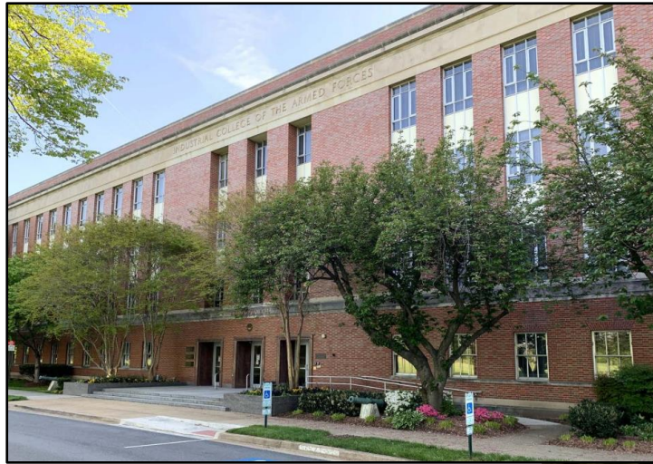
National Defense University Eisenhower Renovation Sep 2022
