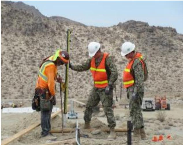
NMCB 3 with Reyes Construction measuring for batter boards onboard NAWS China Lake
