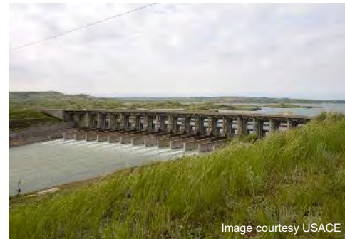
Dam Plunge Pool Repairs Fort Peck, MT
