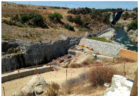
Folsom Dam Auxiliary Spillway Folsom, CA
