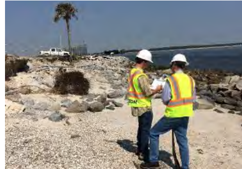
Shoreline Erosion Repair Investigation NS Mayport, FL
