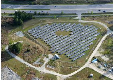
Sustainable Energy/ Photovoltaic D-B Construction MCB Camp Lejeune, NC
