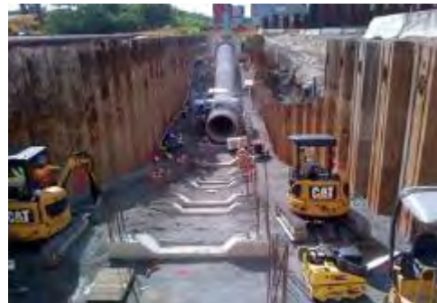
Rio Puerto Nuevo Flood Control San Juan, Puerto Rico
