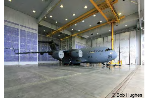
C-17 Corrosion Control Hangar Joint Base Pearl Harbor-Hickam, HI
