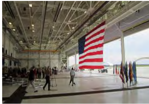
F-35 Hangar & Aircraft Apron MCAS Beaufort, SC
