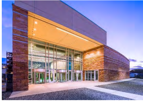
U.S. Army Pacific Mission Command Facility Fort Shafter, HI
