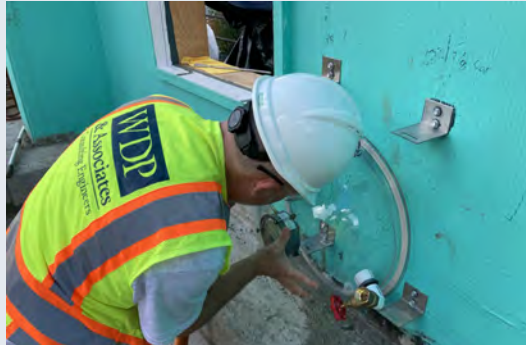
Air Leakage Testing
