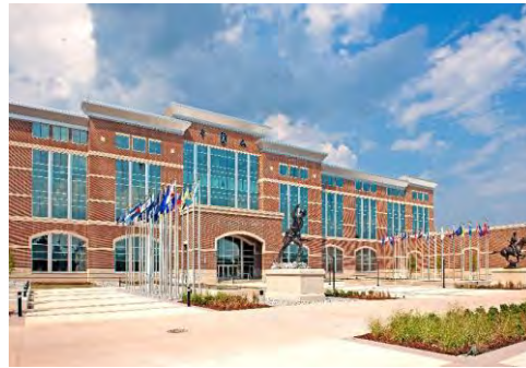
U.S. Army Maneuver Center of Excellence Renovation Fort Benning, GA
