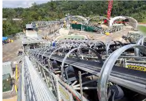
Chickamauga Lock Replacement Chattanooga, TN
