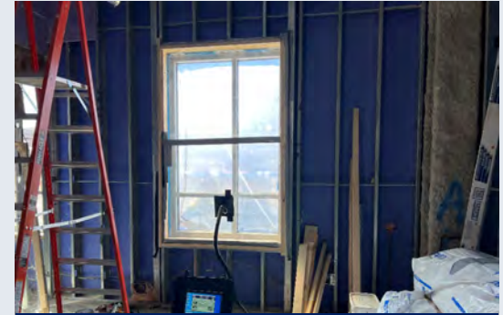
Window Leak Testing
