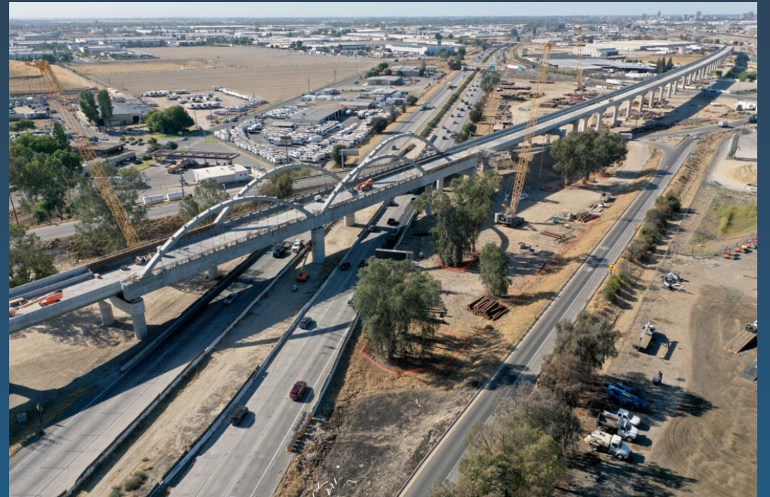
California High-Speed Rail at SR 99 (Fresno, CA)
