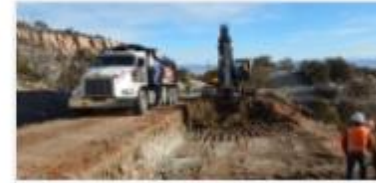
Major Construction Division (MCD)
