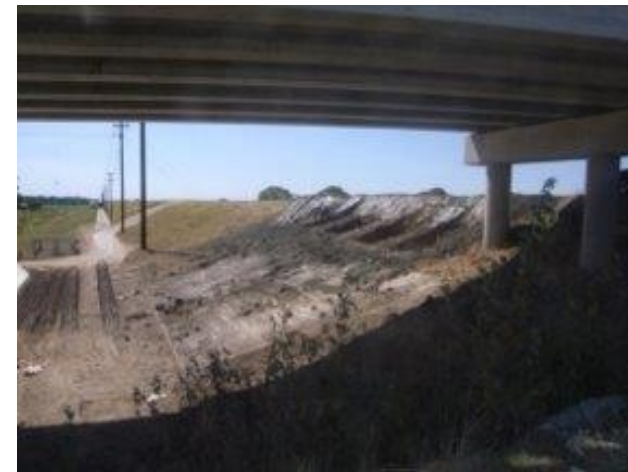
Levee raises and improvements
