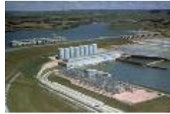
Fort Randall Powerhouse
