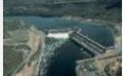
Chief Joseph Powerhouse
