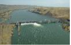
John Day Powerhouse
