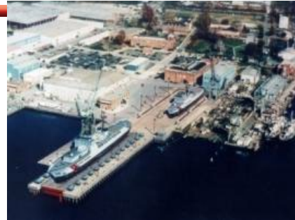
Industrial Facilities & Bases
