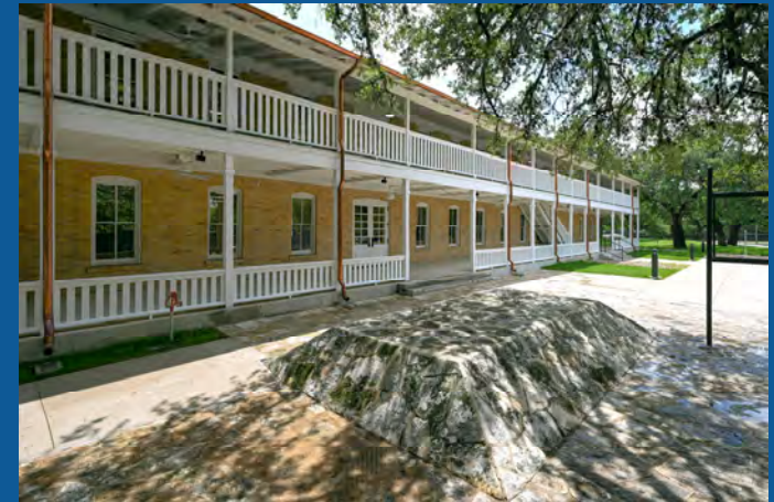
Texas Military Department – Maintenance Renovations
