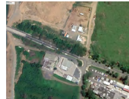
Rio De La Plata Flood Control Project - Utility Relocations (USACE Jacksonville)
