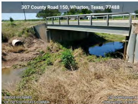
Wharton Levee System (USACE Fort Worth)
