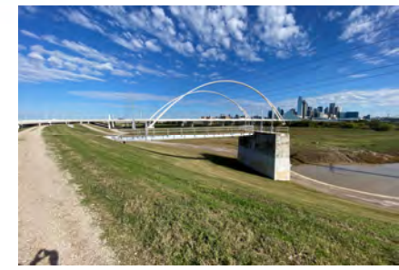
Dallas Floodway Levee Raise and Slope Flattening (USACE Fort Worth)
