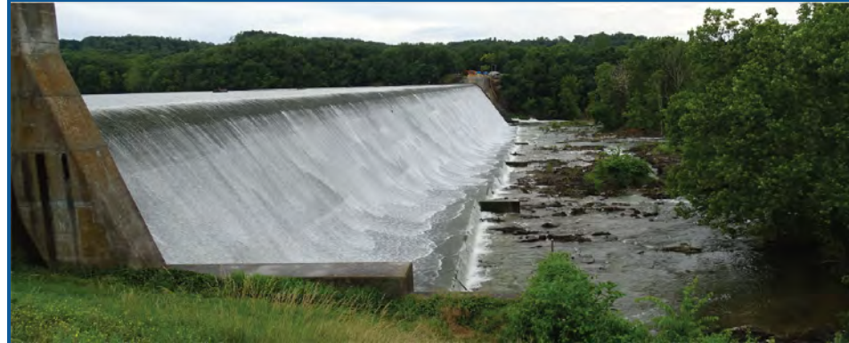
City of Tulsa - Eucha Dam Anchoring
