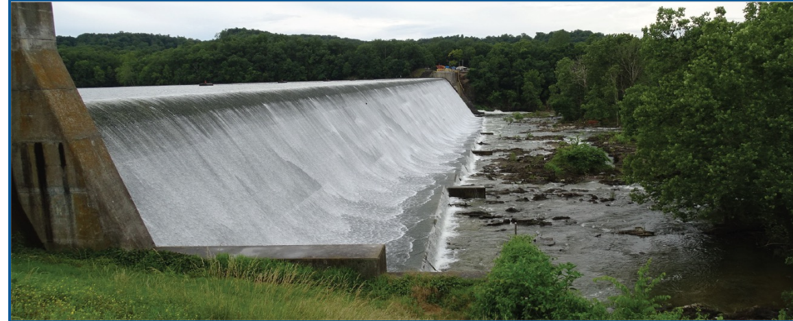
City of Tulsa, Eucha Dam Anchoring
