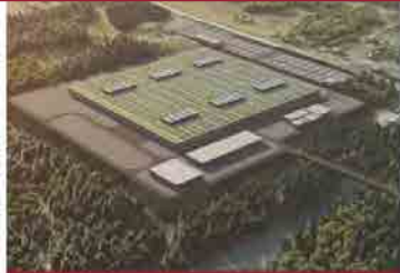
BMW Electric Vehicle Battery Plant Woodruff, SC
