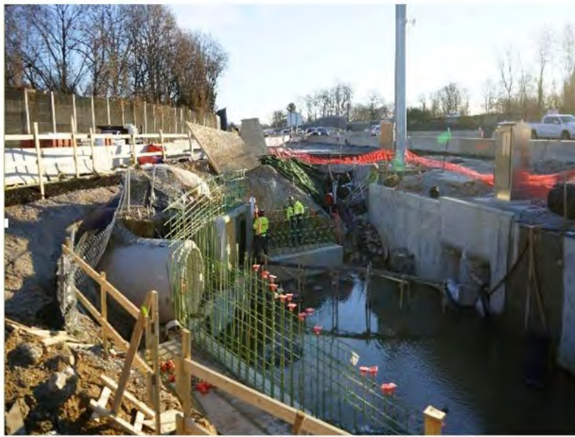
CAST IN PLACE BOX CULVERTS
