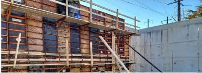
CAST IN PLACE WALLS
