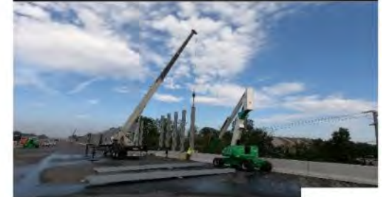
SOUND WALLS INSTALL
