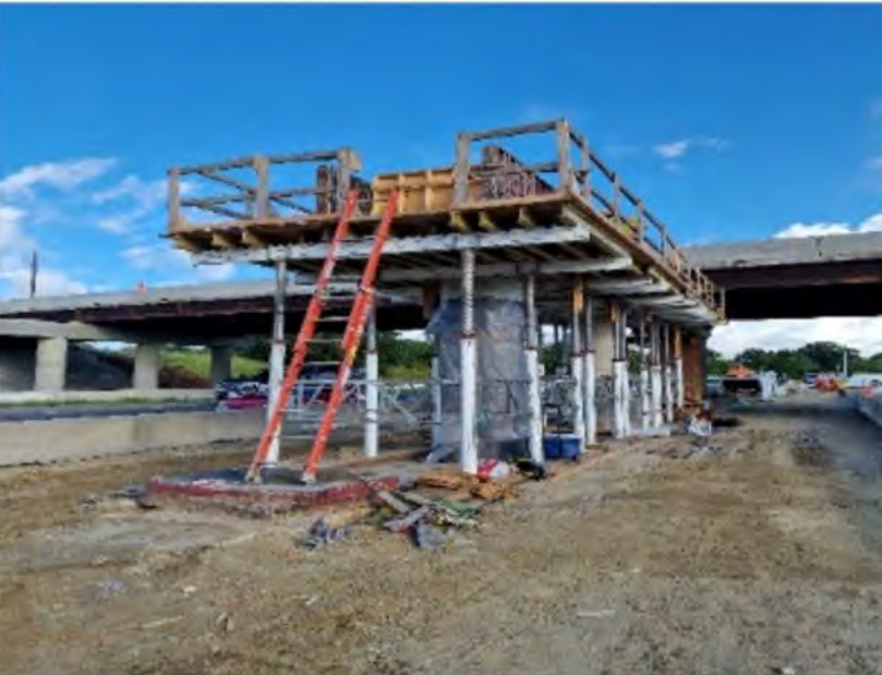
FOOTINGS, COLUMNS AND PIERS
