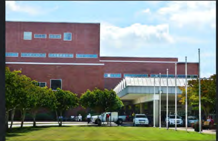
Community Living Center Expansion and Renovation Hunter Holmes McGuire VA Medical Center
