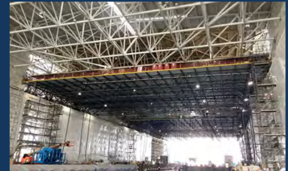
Kings Bay Dry Dock Renovation
