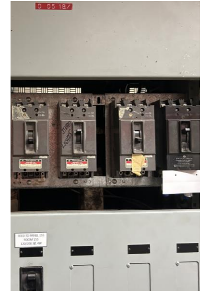
Bagley Lab HVAC Upgrade
